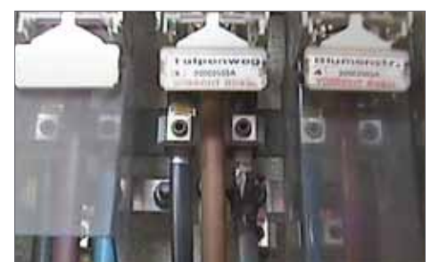
This connector has become resistive due to loosening and corrosion. This can be easily remedied by opening, cleaning and reassembling the connector.
